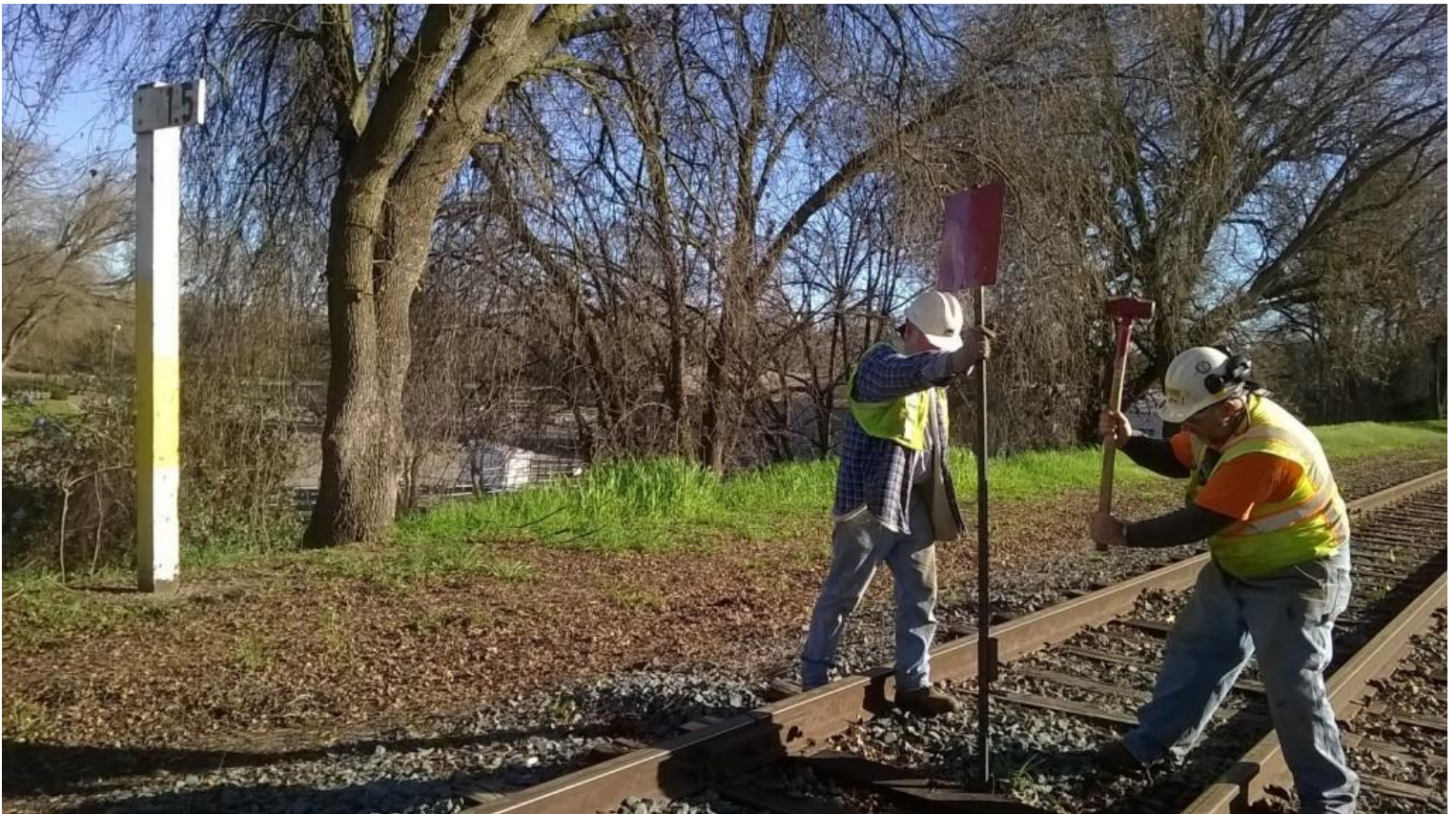
But, Train Order 103 remains in effect. Mike M. and Mike F. plant the RED FLAG at Mile Post 1.5
