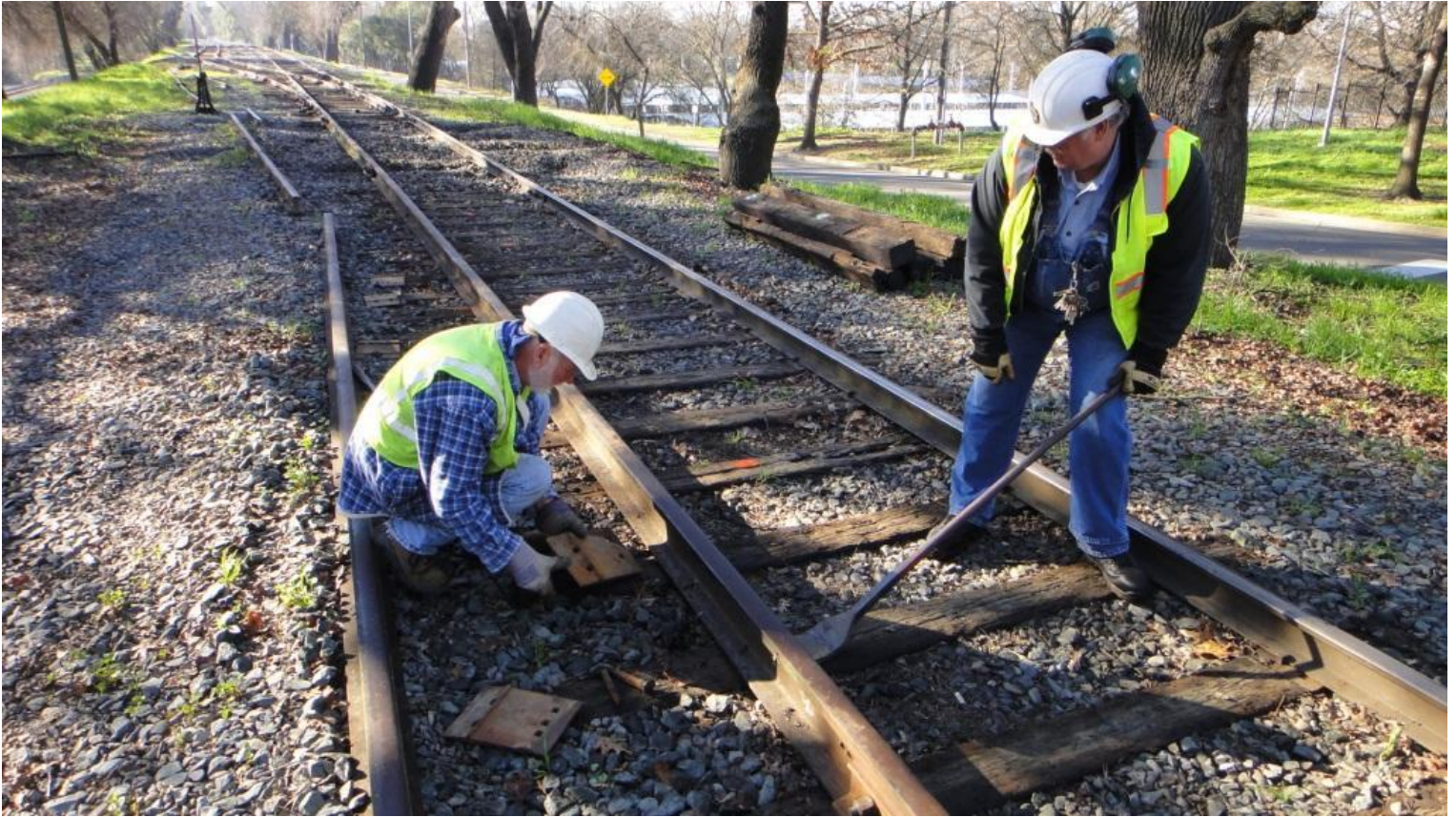
Chris C. nips-up the rail as Mike M. places a tie-plate
