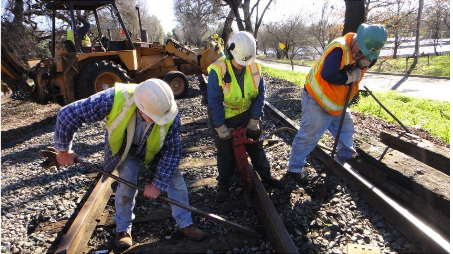
Then Heather comes in and spikes it in gauge with Mike M. and Al nipping-up the rail and tie
