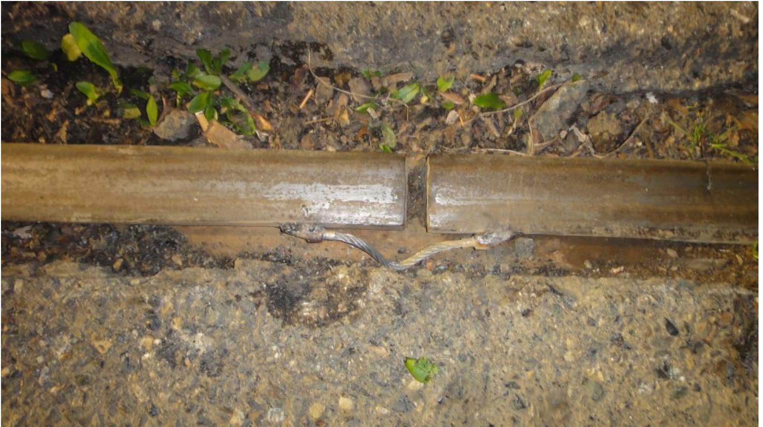
The repaired bond
