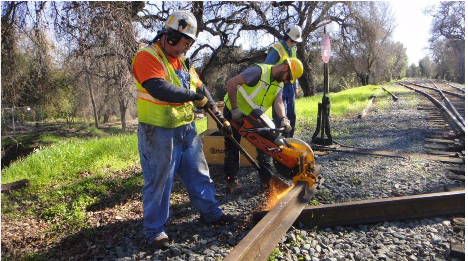
Mike F. deploys a shovel as a spark-shield as Chris M. slices through the rail with the rail-saw
