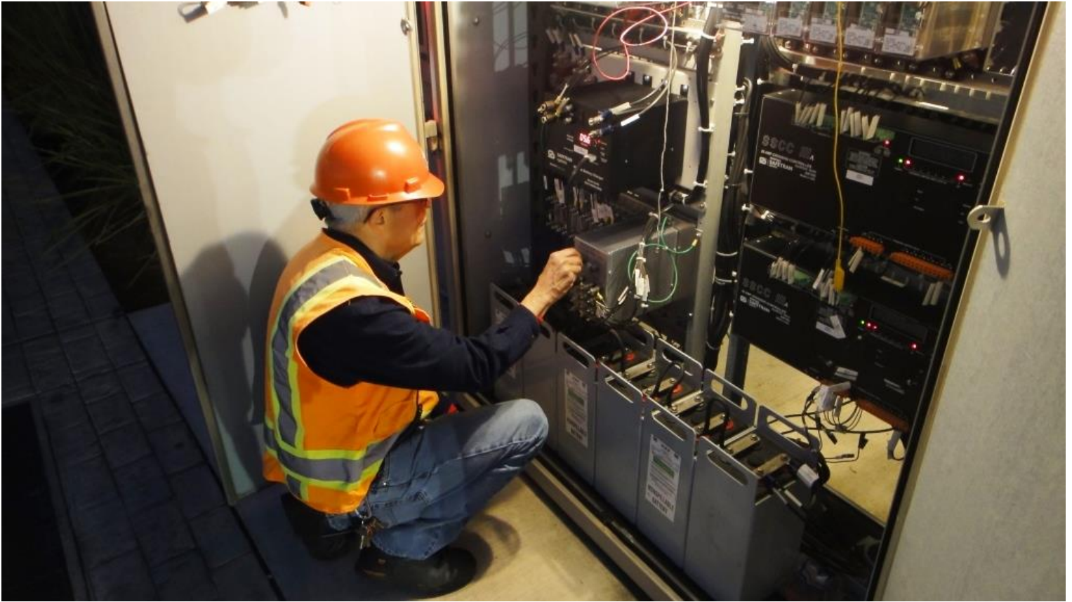
Dale "re-energizes" the Capitol Mall circuit
