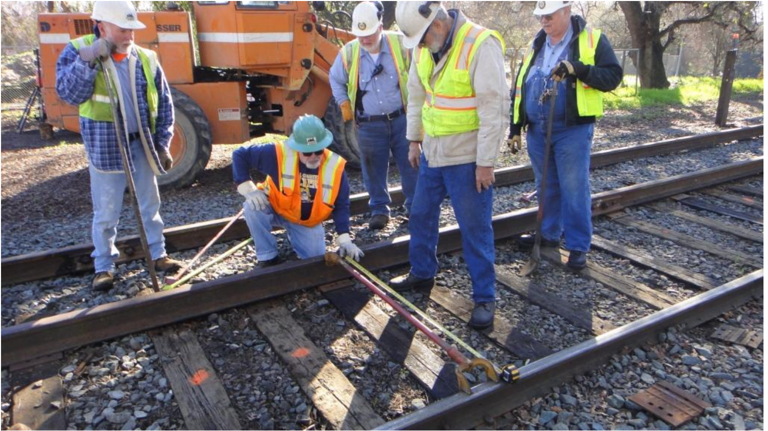
Mike M., Al, Frank, Alan, and Chris C. double check the gauge measurements before setting spikes
