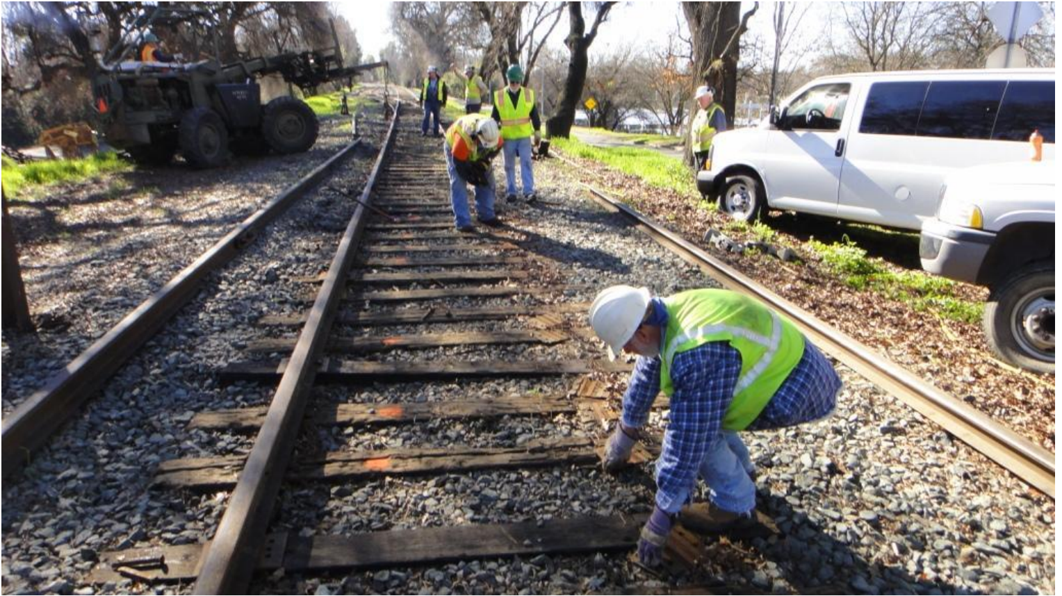
With the old west-rail gone, Mike M and Mike F. collect old 75 lb. rail tie-plates
