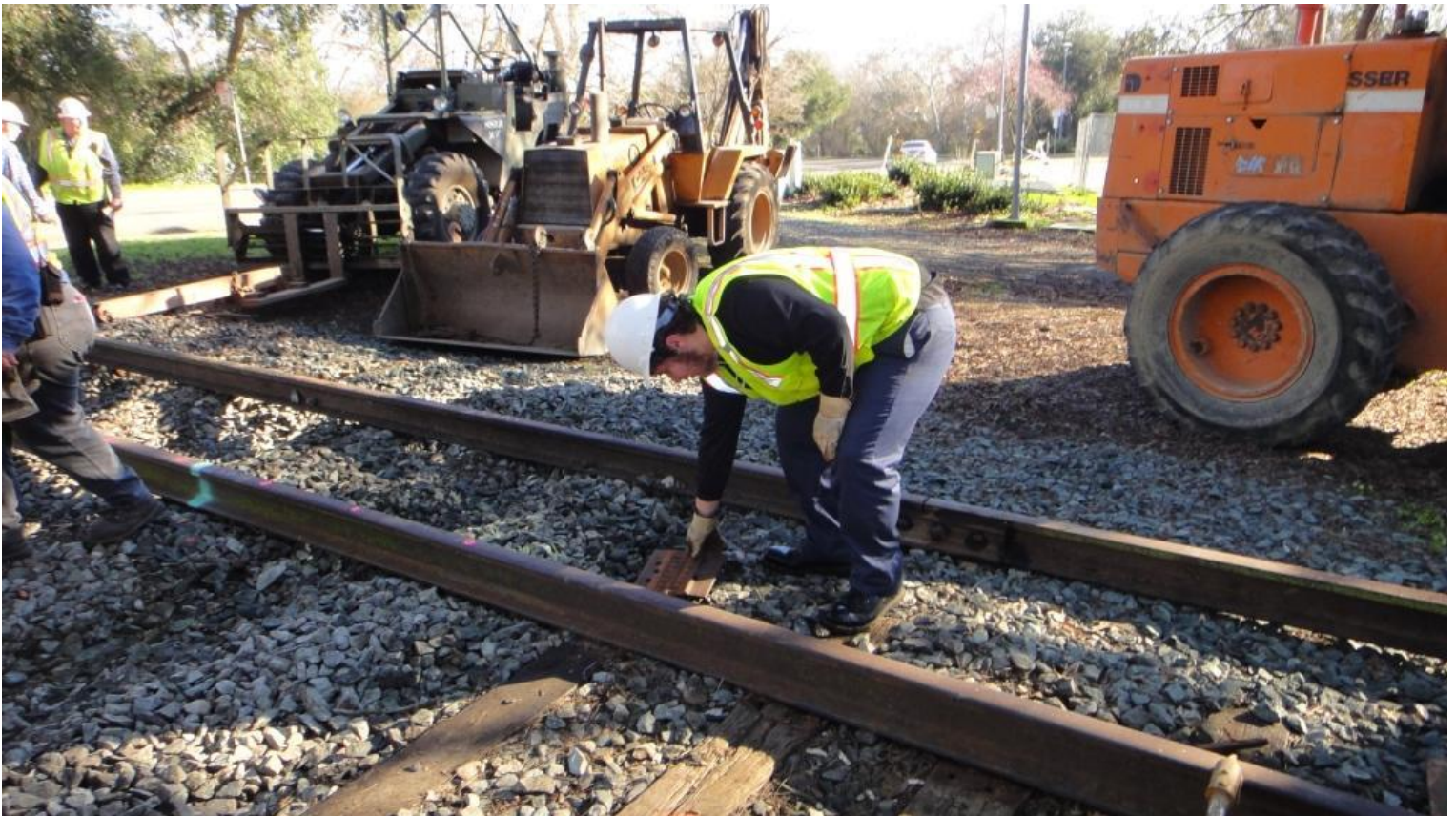
Josh distributing tie-plates for the east-rail
