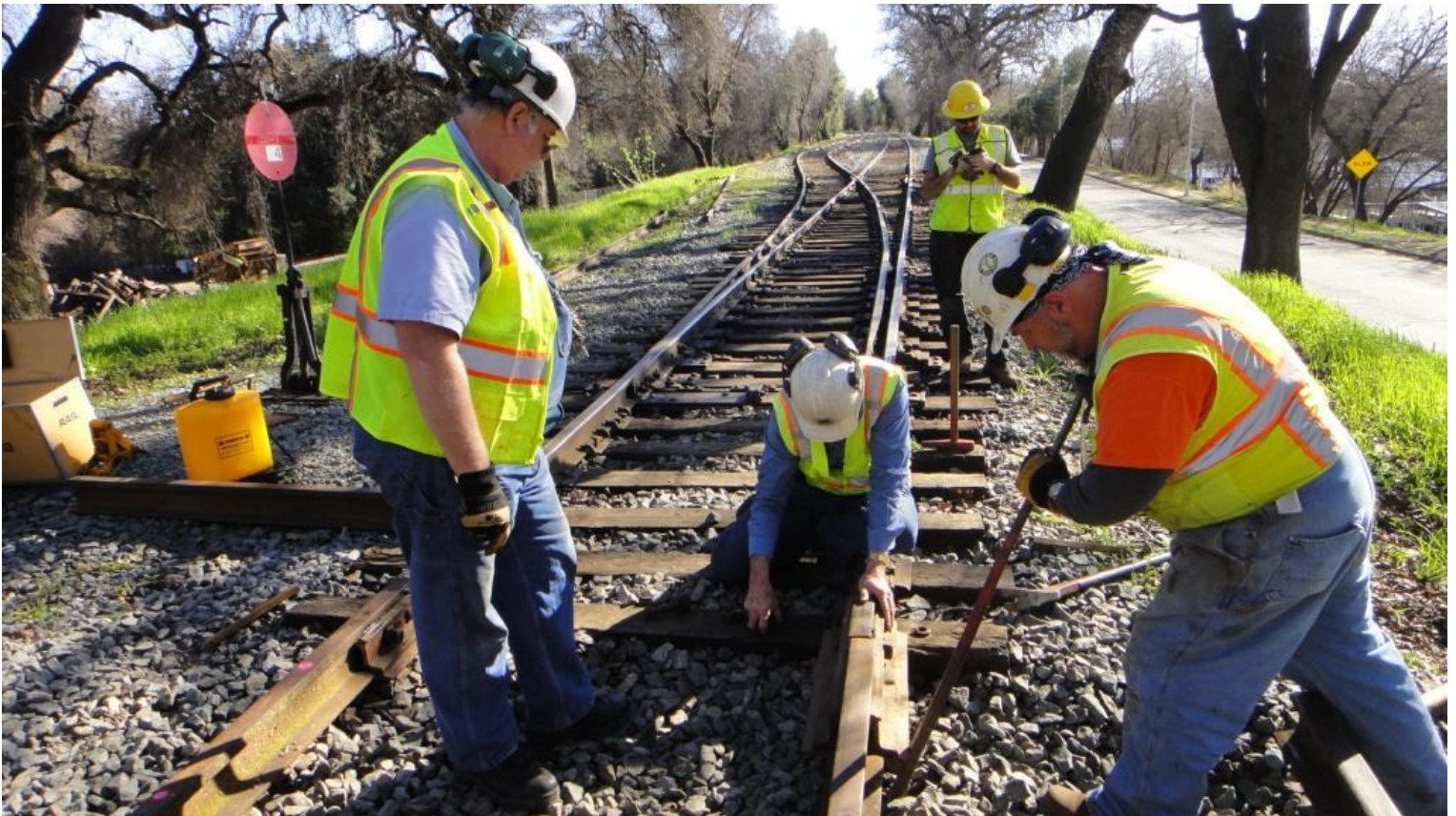
Alan starts the bolts at the comp-joint as Mike F. holds it all together
