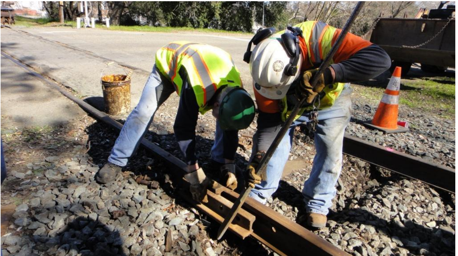
Tom and Mike F. bolt the track together
