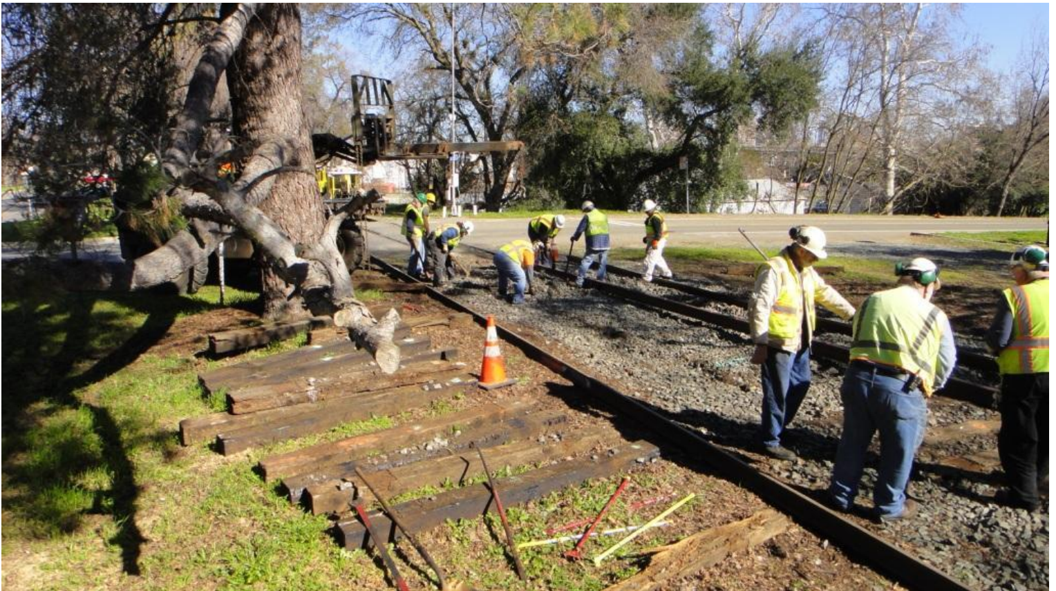
The Team works to dig-out high-spots in the ballast so that the new, taller west-rail will line up with the track at Front Street
