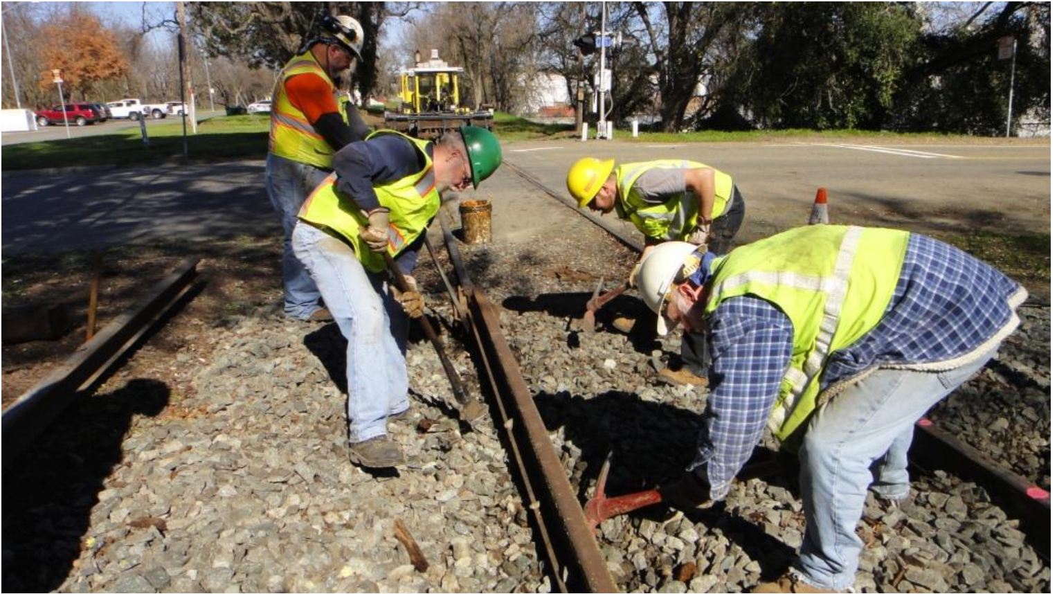
Mike F., Tom, Chris M., and Mike M. cut-down high-spots in the ballast in order to lower the new west rail to align with the track
