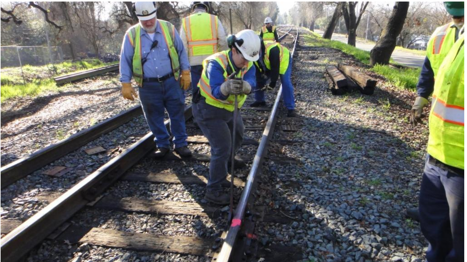
Heather loosens a bolt at a joint designated to be taken apart on the west-rail
