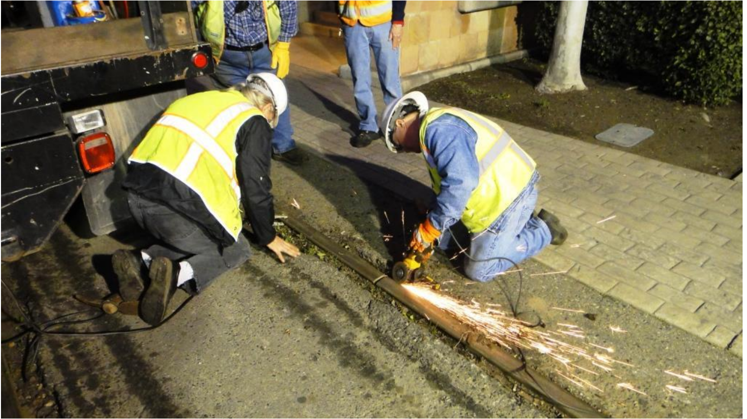
Working under the lights, Fred and Mike H. prep the rail for welding
