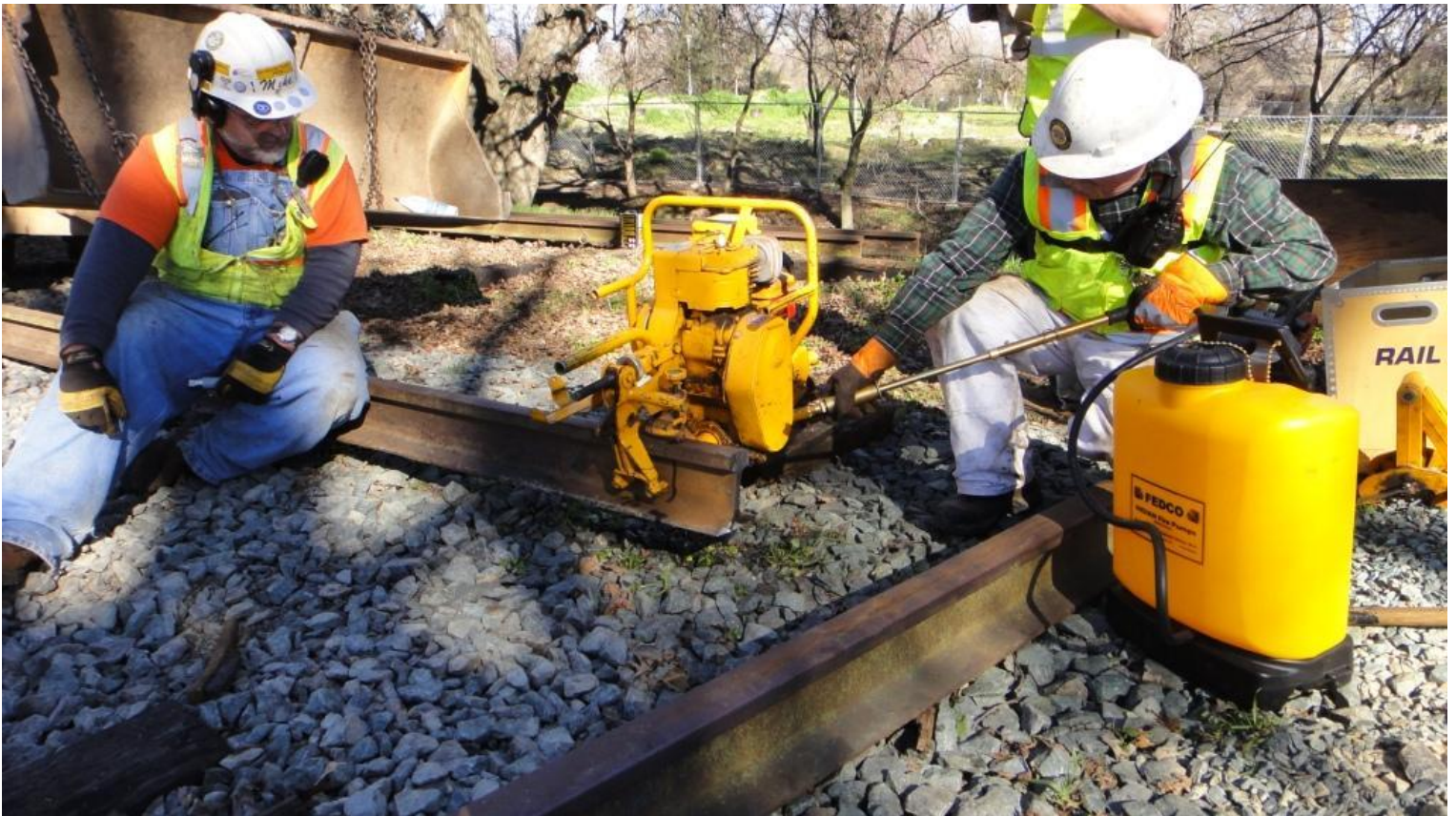
The rail-drill cuts the first bolt hole as Mike H. cools the drill-bit with a stream of water
