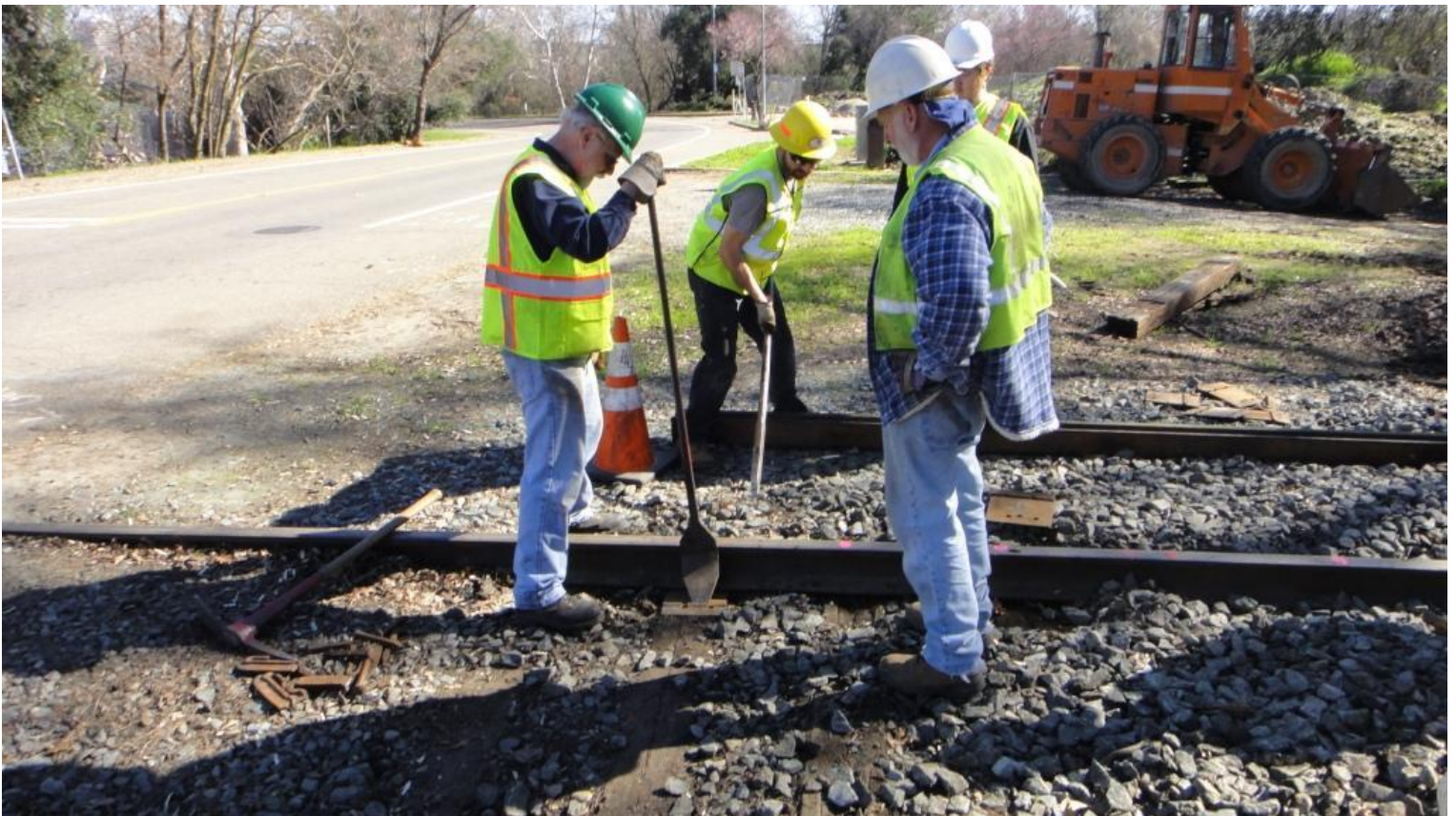
Tom and Chris M. pry-out tie-plates
