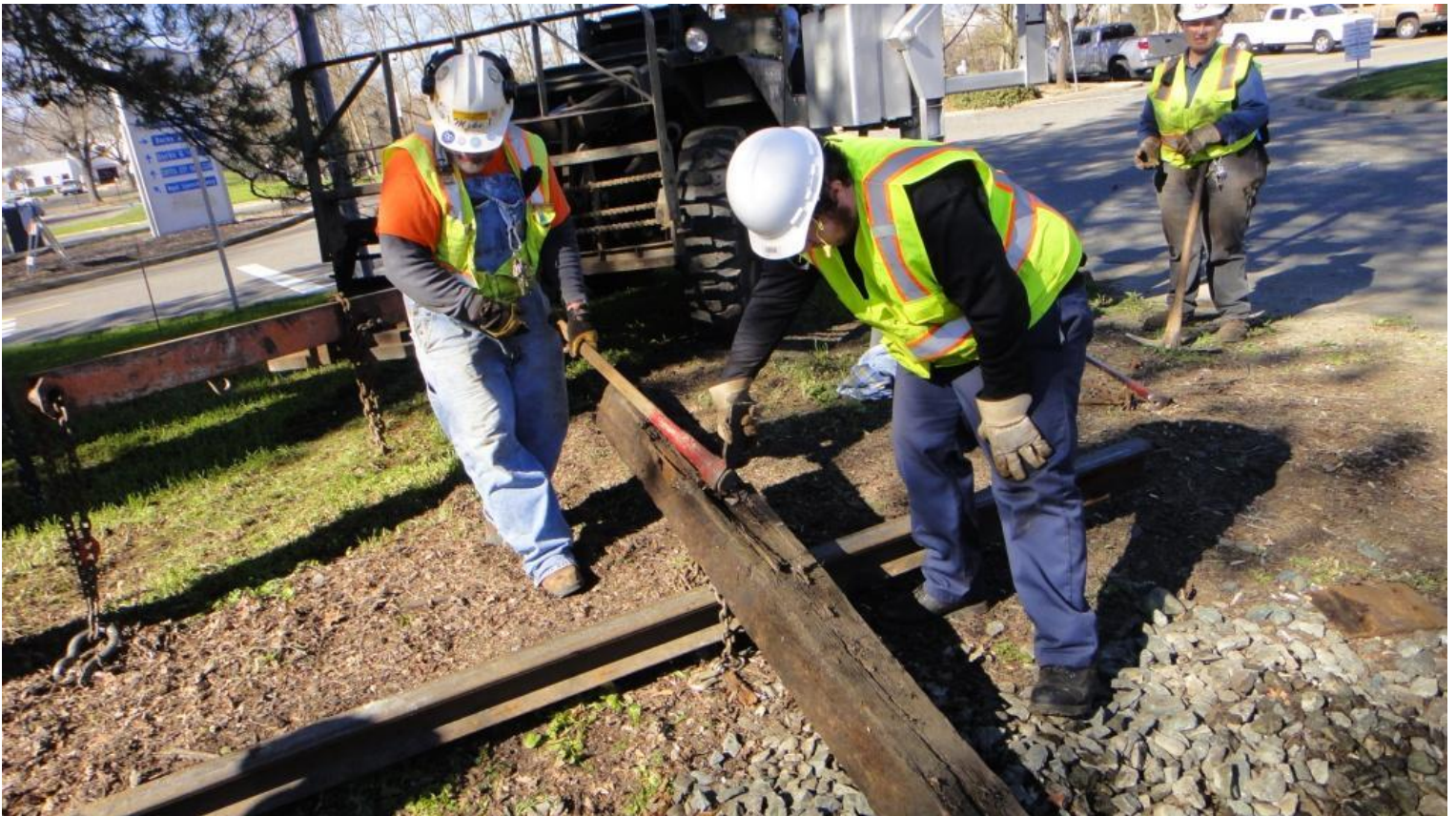
Mike F. and Josh remove a rotten old tie
