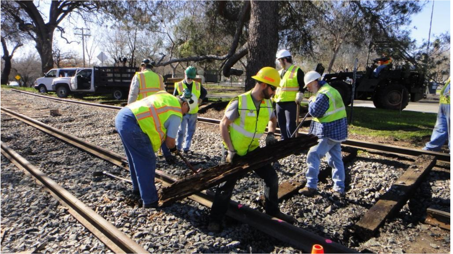
Chris M. carries away the remnant of a tie
