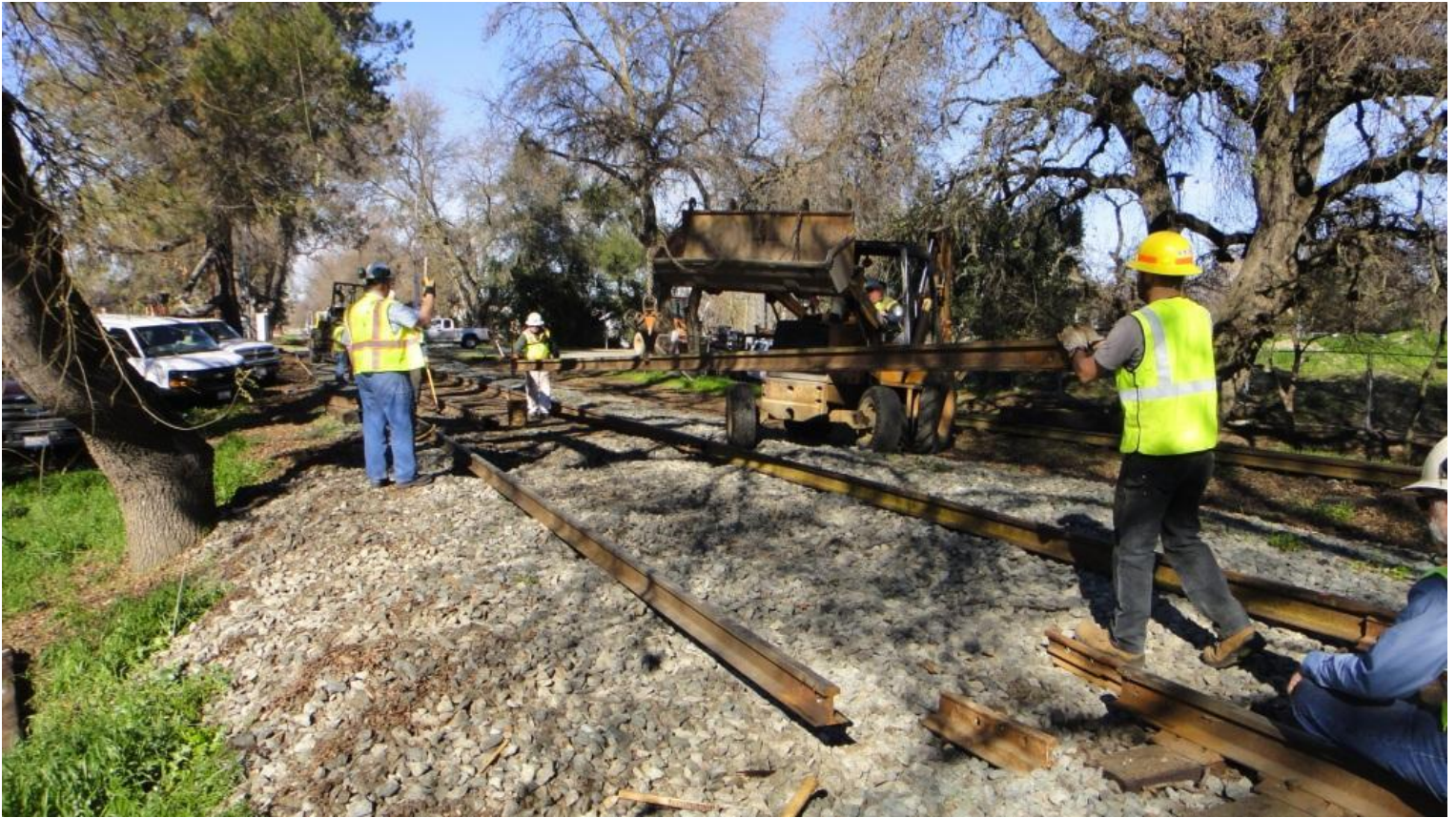
Cut and drilled, the final stick of rail is guided into place
