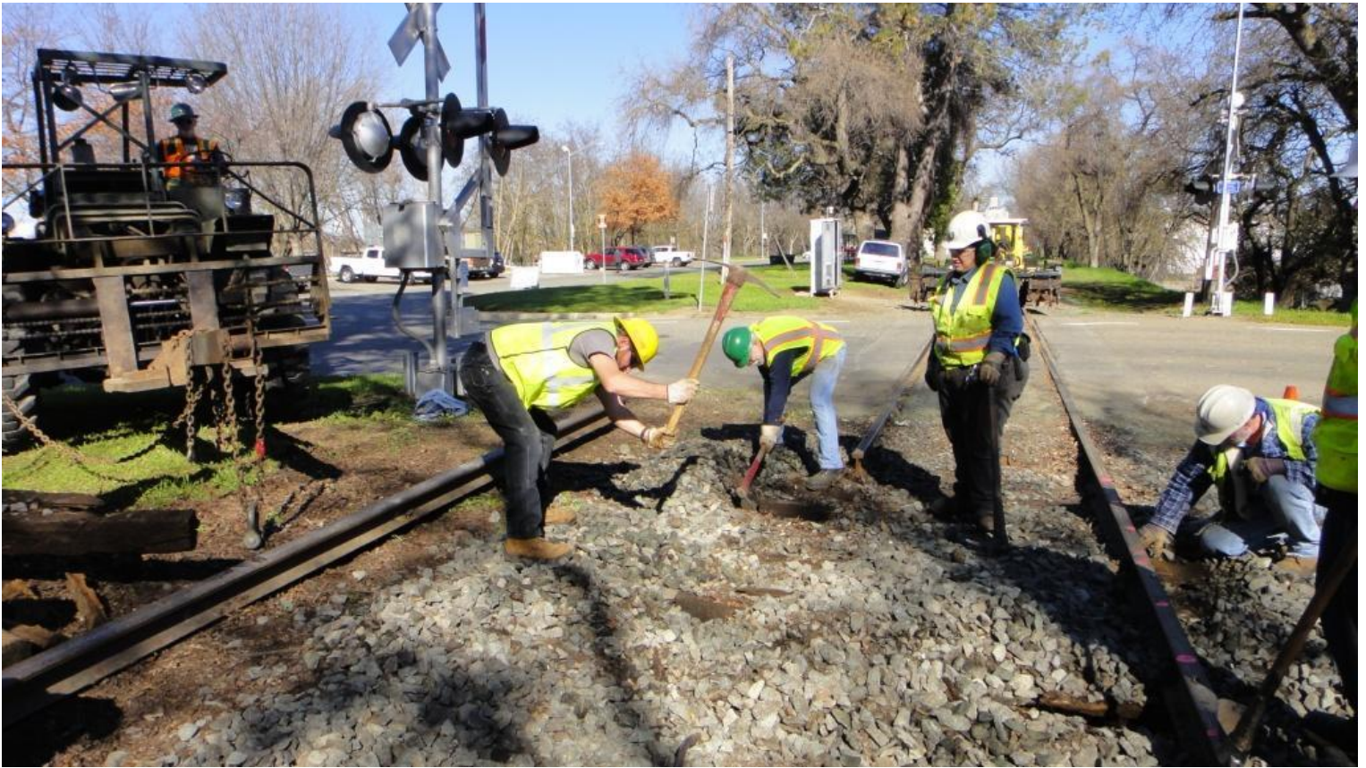
Chris M., Tom, and Heather dig-out the ties at the north end
