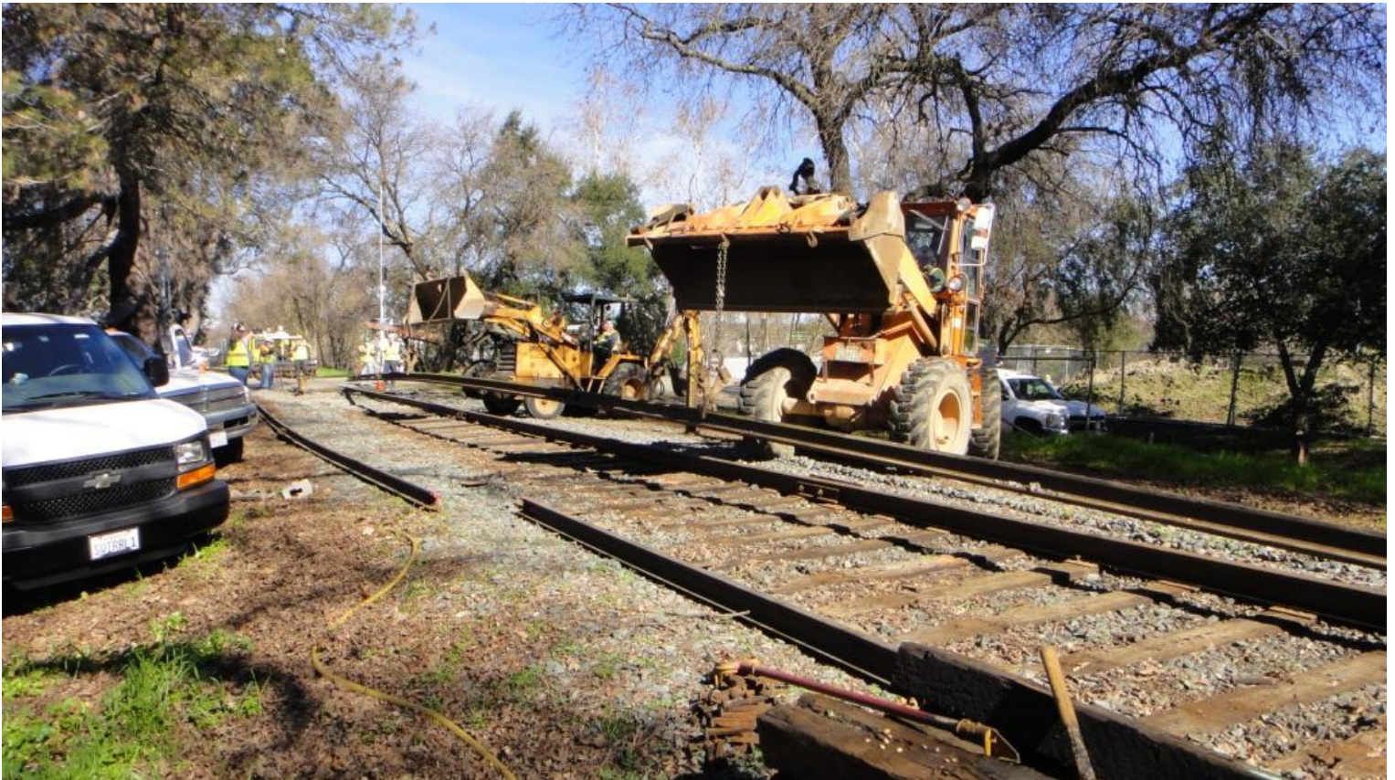
The new west-rail arrives on site...
