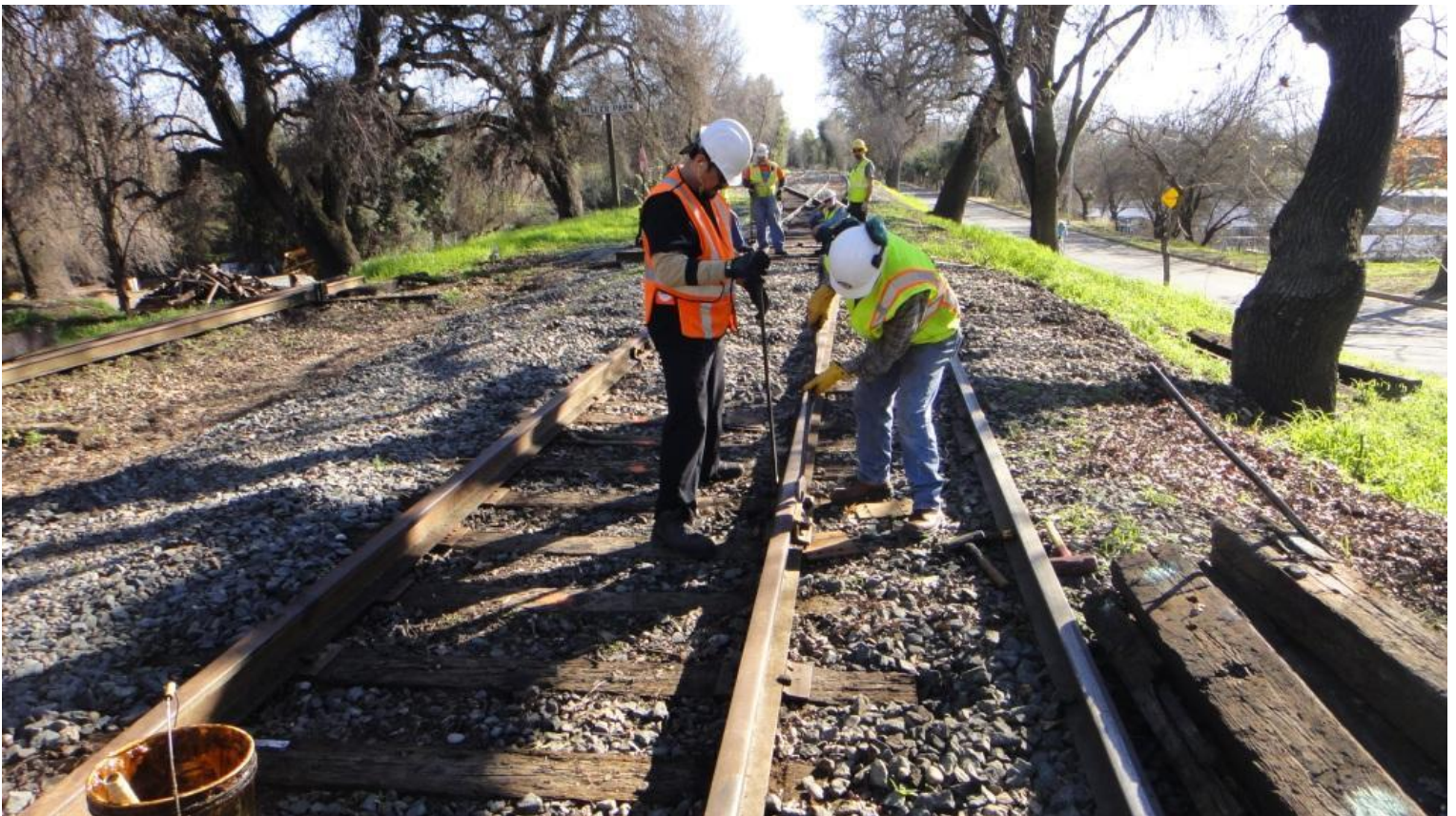
Jose and Mike W. tighten the last bolts on the west rail
