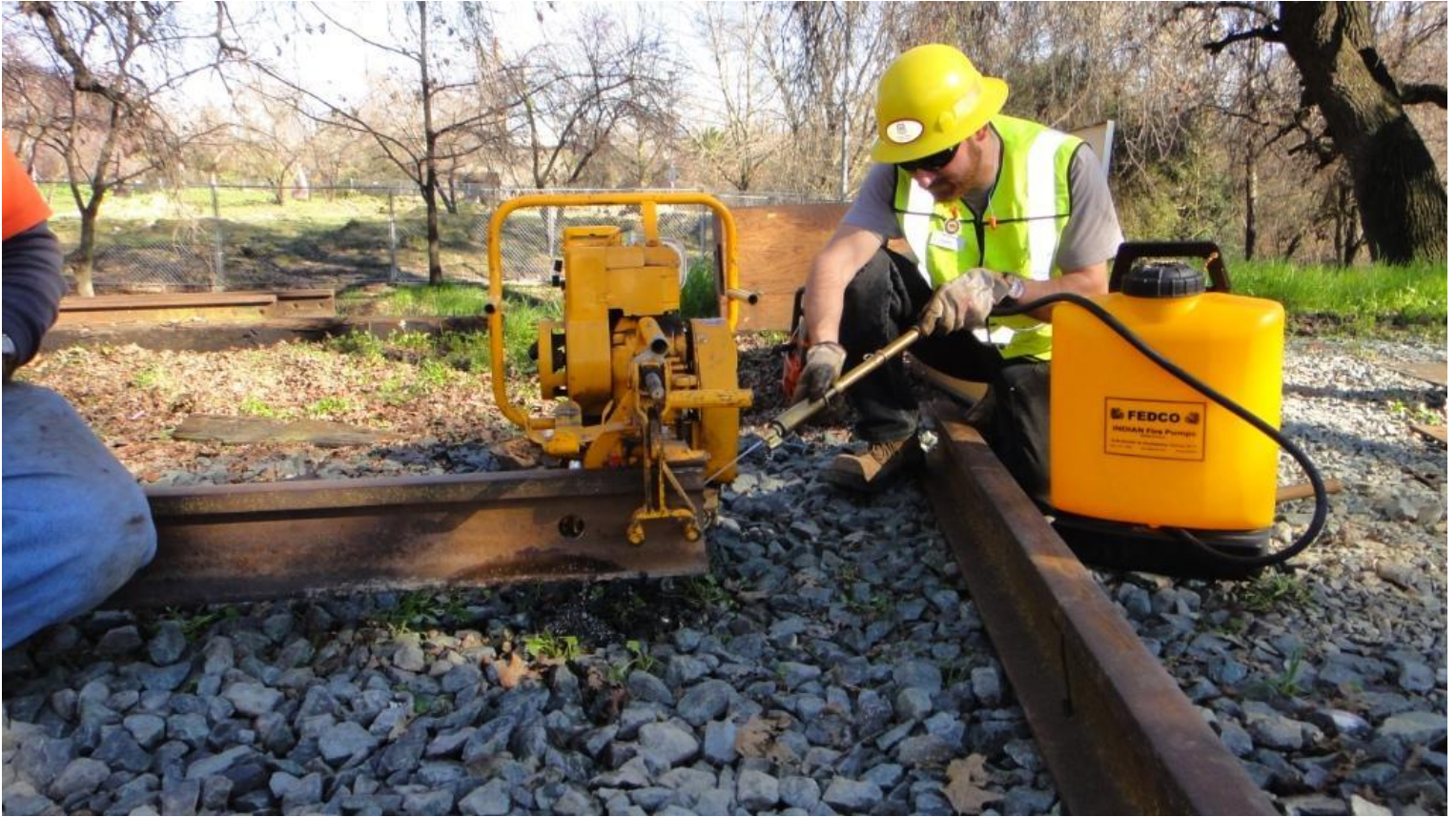
Now it's time to drill the second bolt-hole. Chris M. keeps the drill-bit cool
