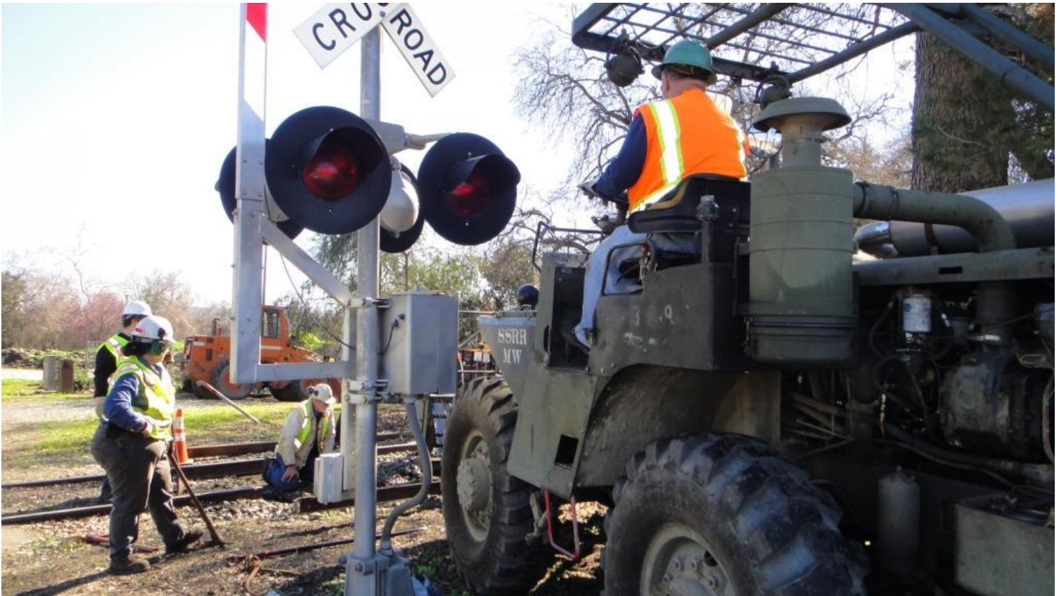
Now that's a tight fit – Al maneuvers the Big Green Machine through a very tight corridor...
